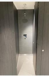
Unity Full Height SGL shower cubicles were specified for the changing rooms. The full height floor to ceiling cubicles are ideal for creating complete privacy. The doors and panels are manufactured using Solid Grade Laminate (SGL), ensuring the shower cubicles are completely water resistant and hardwearing.
